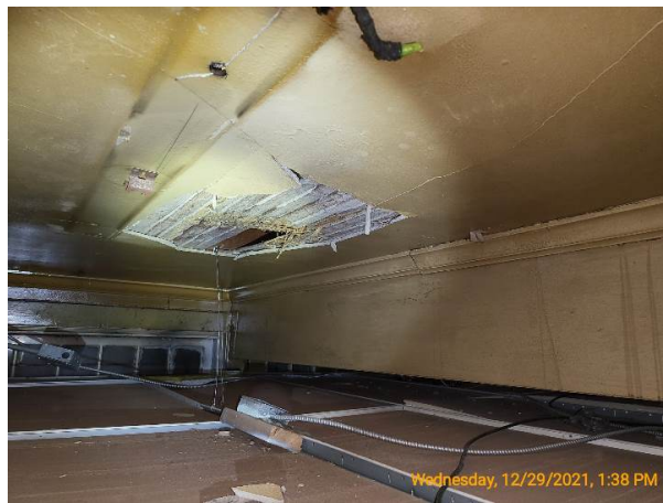
Plaster ceiling covers most of the right half of 714
