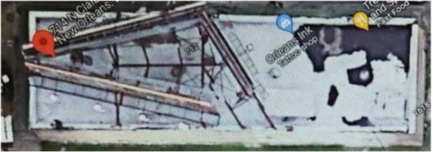
Overhead view - Building appears to sit on the property lines
