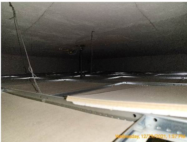
Plaster covers the ceiling joists
