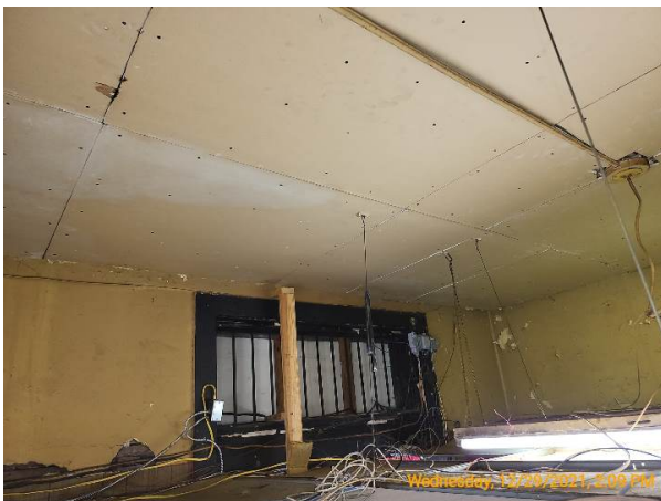
Sheetrock across the beams above the first floor
