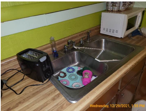
Severely low water flow
