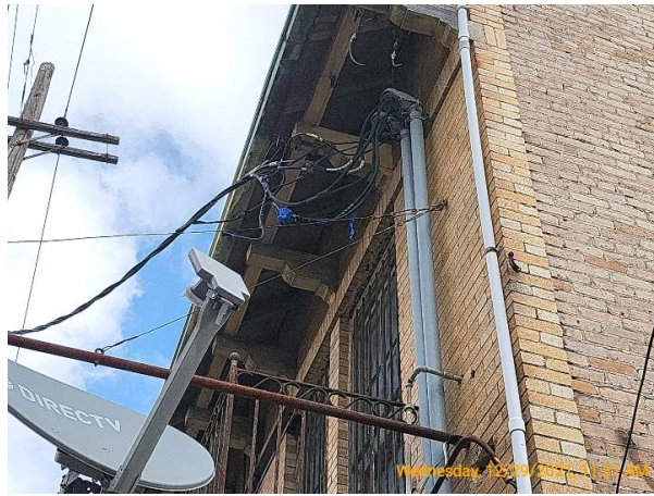
Main electrical entry point at the right front corner
