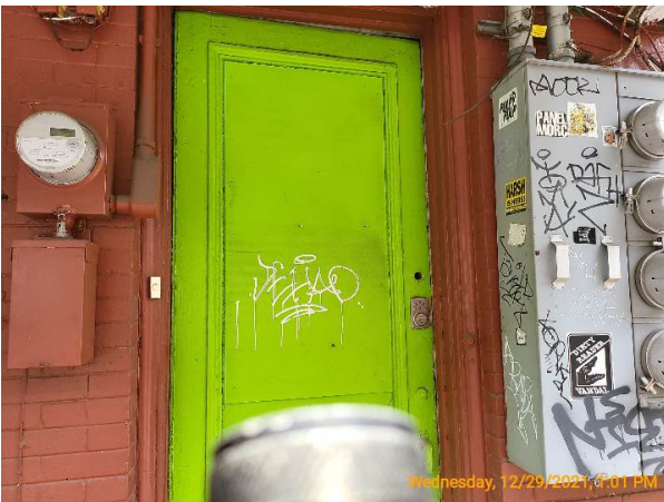
712 North Claiborne is the second floor front unit
