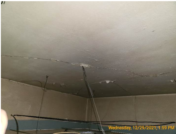
Plaster ceilings above the drop down on the second floor of 1620
