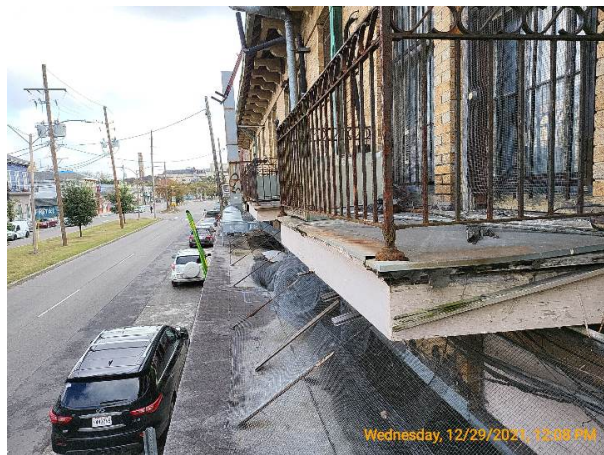
9 balconies in all
