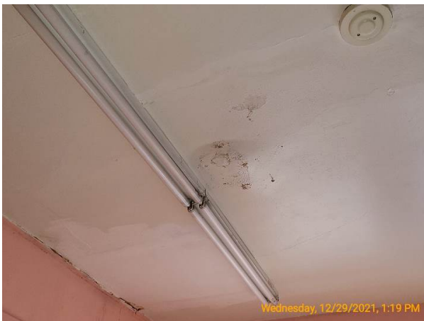
Evidence of active leakage at a left side bedroom and between the two bedrooms
