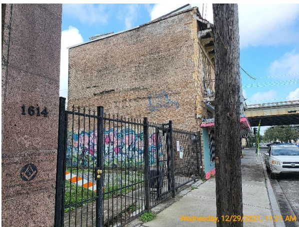
The rear of the building
