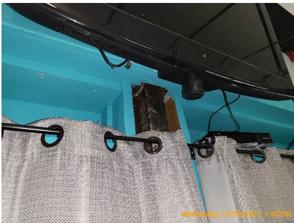
Steel post at the central front wall supporting the beam in 714
