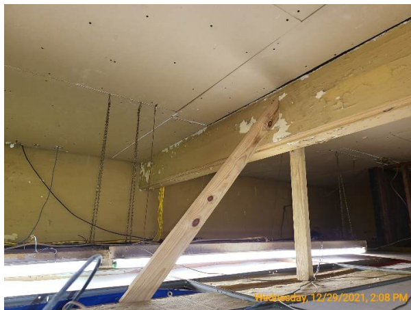
Central beam across the first floor appears functional
