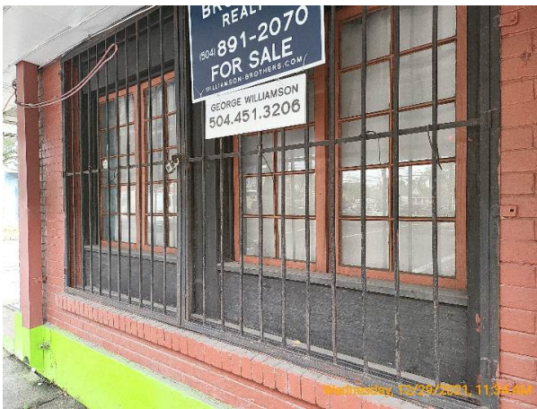
Burglar bars noted on most windows and doors
