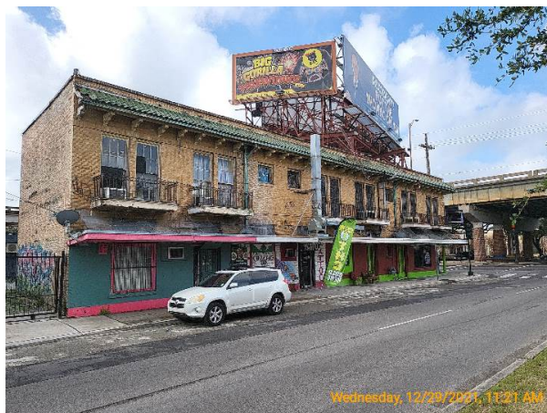
The left side of the building
