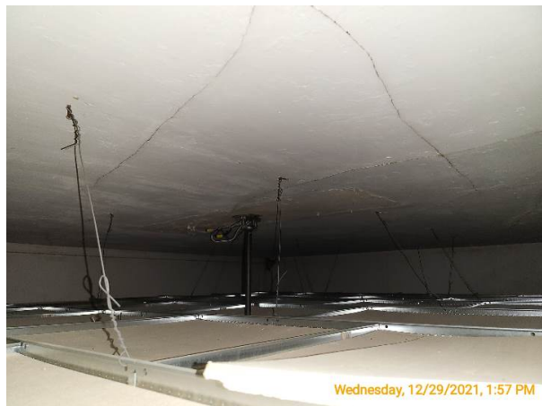
Plaster covers the ceiling joists
