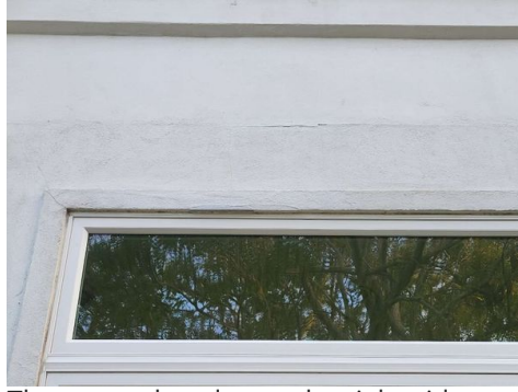
The accent band over the right side rear window is damaged
