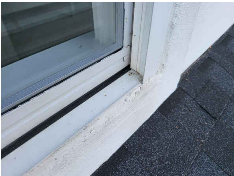
Older windows with miter joints
