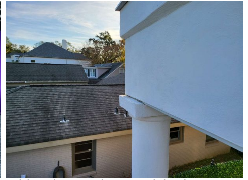
Add sealant to the top of the front porch capitals
